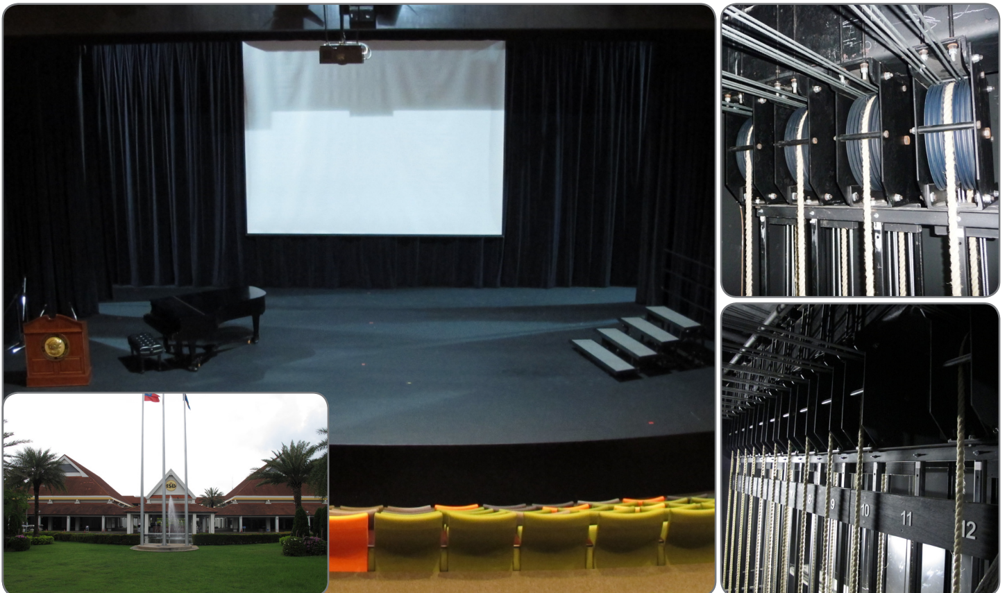
The stage of the ISB's Cultural Centre dressed with curtains and a cyclorama by J&C Joel (Above). A complete rigging system was also provided (right)
